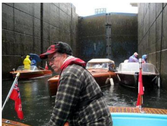
A conventional lock is a watertight chamber with a watertight gate at each end. If the valves in the lower gate are opened and those in the upper gate remain closed, the water runs out. Boats inside the lock are thereby lowered. When the valves in the lower gate are closed and those in the upper one are opened, the lock fills with water and boats are raised.
